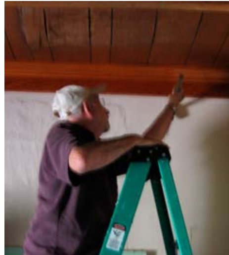
Bruce Baker checks out the modern paneled ceiling in the kitchen.
