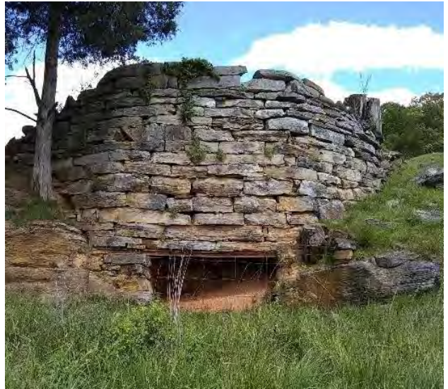
Lime kiln, Reeves Road, Augusta County.
